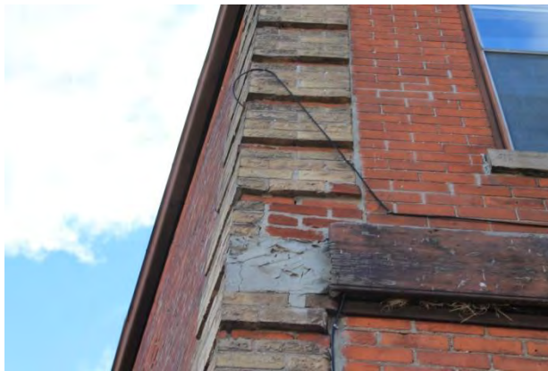
Figure 83 & 84 – (left) Detail of west elevation quoins noting existing incompatible mortar repairs (right) Detail of south elevation quoins noting pitted and weathered brick (Source: MHBC, 2016)
