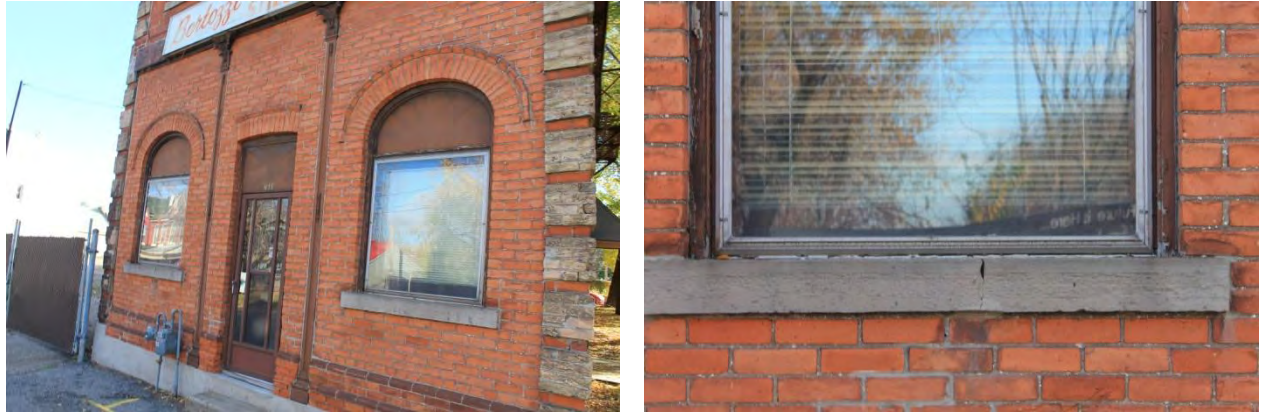
Figures 47 & 48 – (left) View of west elevation of Building 'A-1', first storey door and window openings (right) Detail view of west elevation of Building 'A-1' textured stone sill (Source: MHBC, 2016).
