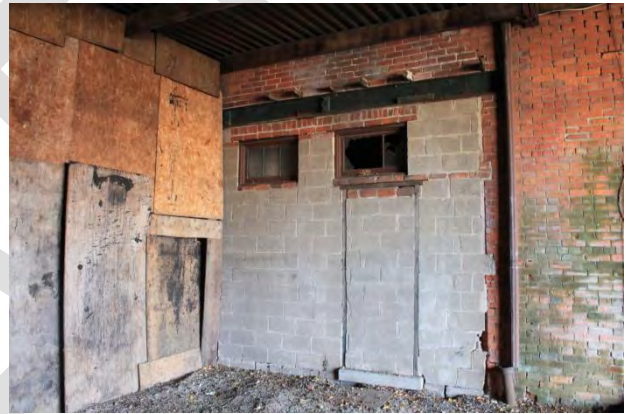
Figures 31 & 32 – (left) View of north elevation of Building 'A-2', looking south-east towards person door and bricked-over passage way or carriage way (right) Detail view of bricked-over passage way at north elevation of Building 'A-2' looking south-east under sheet metal structure. (Source: MHBC, 2016)
