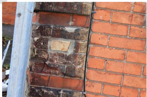
Figure 85 & 86 – (left) Detail of west elevation steel pilasters, noting condition of surrounding masonry (right) Detail of west elevation quoins noting previous incompatible repair work (Source: MHBC, 2016)
