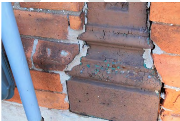
Figure 85 & 86 – (left) Detail of west elevation steel pilasters, noting condition of surrounding masonry (right) Detail of west elevation quoins noting previous incompatible repair work (Source: MHBC, 2016)
