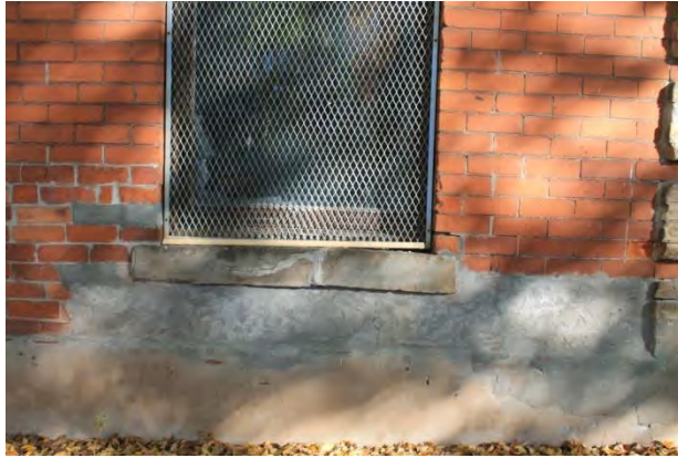
Figure 81 & 82 – (left) Detail of south elevation first storey window noting cracked stone sill (right) Detail of south elevation brick quoins noting failures of previous mortar repairs (Source: MHBC, 2016)
