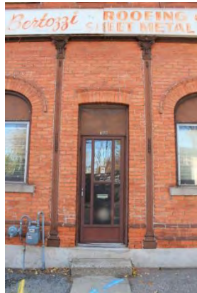
Figures 43 & 44 – (left) View of west elevation of Building 'A-1', first storey doorway and pilasters (right) Detail view of west elevation of Building 'A-1' drip mould above doorway and Corinthian order pilasters (Source: MHBC, 2016).
