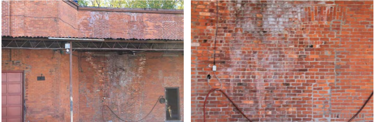
Figure 87 & 88 – (left) View of North elevation, noting efflorescence (white residue) of masonry (right) Detail of North elevation, noting efflorescence (white residue) of masonry (Source: MHBC, 2016)
