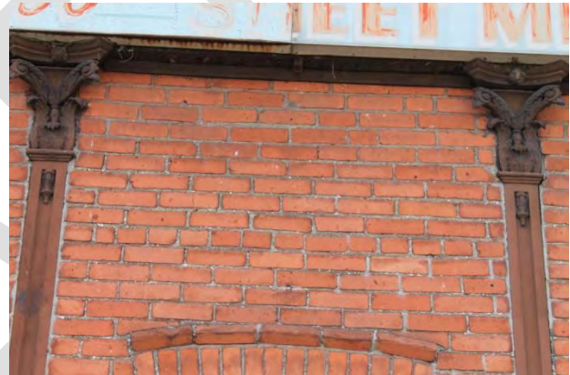
Figures 43 & 44 – (left) View of west elevation of Building 'A-1', first storey doorway and pilasters (right) Detail view of west elevation of Building 'A-1' drip mould above doorway and Corinthian order pilasters (Source: MHBC, 2016).
