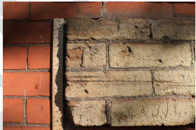
Figure 83 & 84 – (left) Detail of west elevation quoins noting existing incompatible mortar repairs (right) Detail of south elevation quoins noting pitted and weathered brick (Source: MHBC, 2016)
