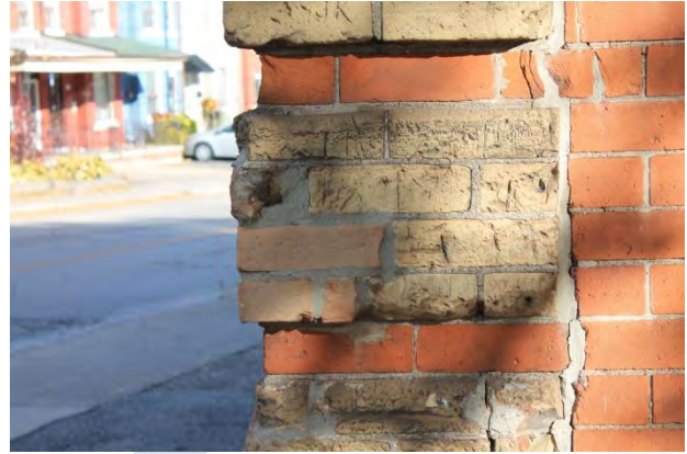
Figure 81 & 82 – (left) Detail of south elevation first storey window noting cracked stone sill (right) Detail of south elevation brick quoins noting failures of previous mortar repairs (Source: MHBC, 2016)
