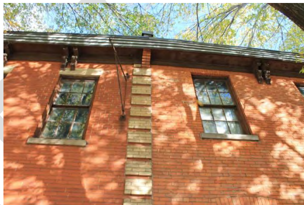
Figures 59 & 60– (left) View of south elevation, second storey windows near intersection of Building 'A-1' and Building 'A-2' (right) View of second storey south elevation, brick quoins dividing Building 'A-1' and Building 'A-2', noting different window styles and paired brackets overlapping windowsills towards western end (Source: MHBC, 2016).
