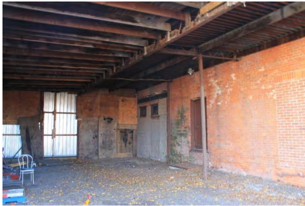
Figures 31 & 32 – (left) View of north elevation of Building 'A-2', looking south-east towards person door and bricked-over passage way or carriage way (right) Detail view of bricked-over passage way at north elevation of Building 'A-2' looking south-east under sheet metal structure. (Source: MHBC, 2016)
